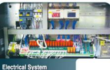
> All new function: PLC data bank. Feed positioning, torque and speed are accurately controlled and perfectly interfaced with the CNC lathe.
