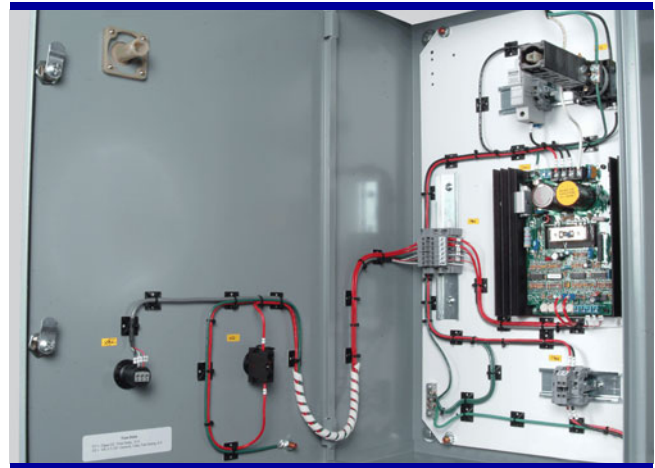
DC motor drive assembled and wired.
