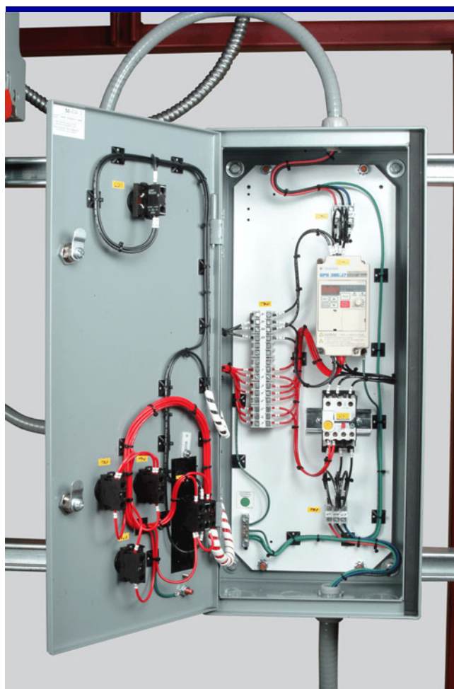
AC motor drive assembled and wired.
