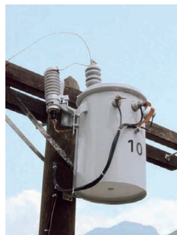
Single hanger bracket one high-voltage bushing self protected unit.
