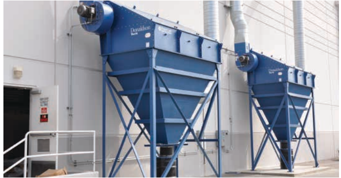
CPC-24 - Paper tissue manufacturing 7,600 cfm (12,910 m 3 /h)
