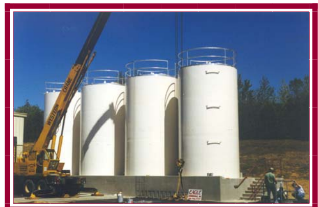
Welded Smooth-Wall Steel Tanks Installation of Welded Tank
