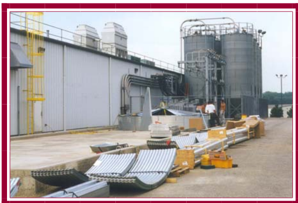
Galvanized Steel, Bolted, Corrugated Tanks Installation of Bolted Tank
